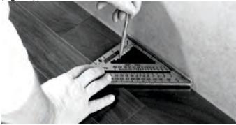
NOTE: Another way to achieve a firm starting point is to screw down a straight length of 1"x3" lumber, or another straight, firm material along the full length
